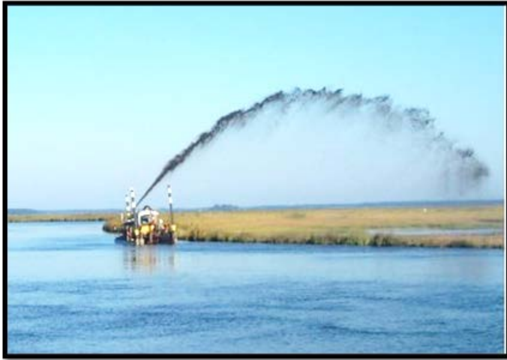
Figure 5-1. High-pressure spray disposal of dredged material (photograph courtesy of Bob Blama, USACE). As effectively demonstrated in Rainey Sanctuary in Vermilion Parish, the primary method of thin-layer placement is to deposit thin layers of sediment by spraying sediment slurry under high pressure over the marsh surface. The technique is essentially a modification of existing hydraulic dredging methods in which sediments are hydraulically dredged, liquefied, and then pumped through a high-pressure spray nozzle.
